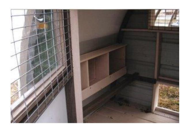
A right side view from the door of the chicken house. Right side you will find a roost pole for the chickens, solid enclosed floor, insulated ceiling, trap door to the outside pen and window view to the outside enclosed run pen.
